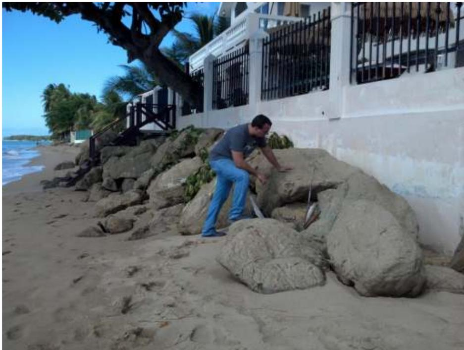
**A10: Sea wall rocks to control erosion. Photo: P. Mejías.**
